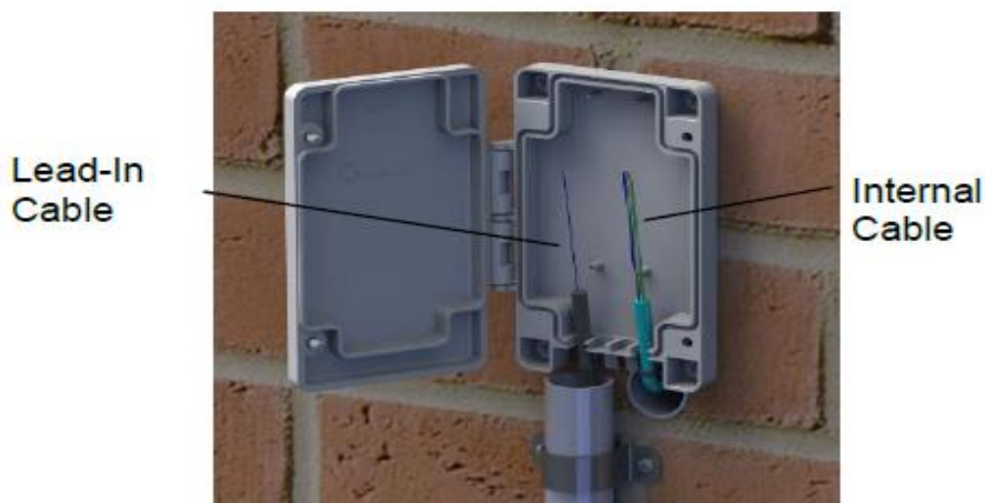
Figure 23. nbn compact NTD with unterminated cables (only white conduit and saddles allowed)
