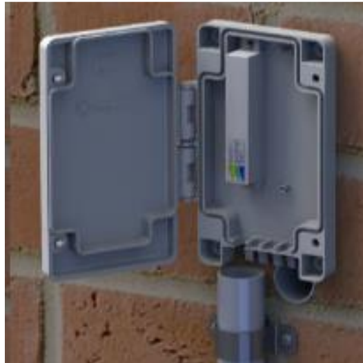
Figure 24. nbn NTD with VDSL2 centralised filter installed (only white conduit and saddles allowed)
